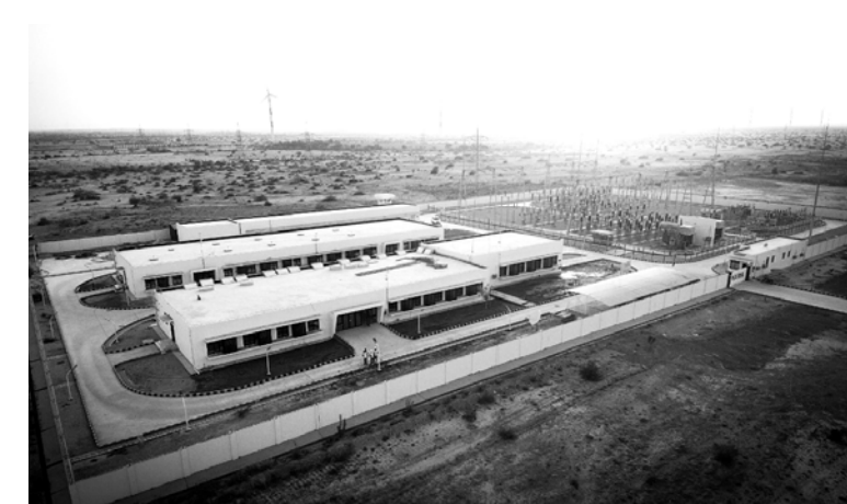
Hawa operating facility, Jhimpir, Pakistan
