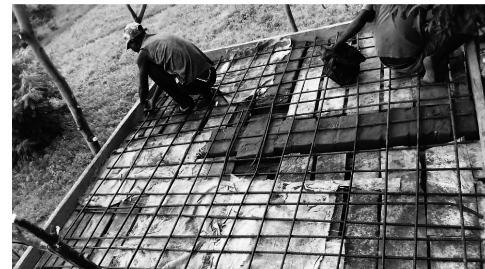
Construction of water tank support base, Namanda Primary School, Salima, Malawi
