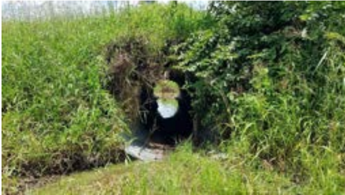
Culvert 1: 673255.68 m E , 8402690.36 m S
